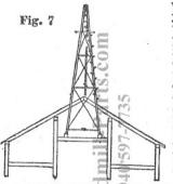
weh as if it were erected over your well, or if your well is near where you wish your machines placed you can erect the mill near the well, or at some convenient point between the well and where machines are to be located, and the machines can be operated by pulleys and line shafting extending from mill to barn, or wherever machines may be. The power windmill is never erected directly over the pump, the pump never being nearer than just outside the tower.
